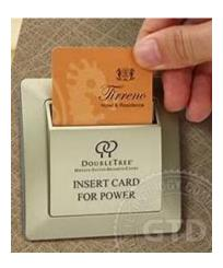
Having a facility for the "Hired rooms" for using the card system to prevent lights and heating being left running when not in use - this would save unnecessary running costs and could be used in conjunction with the keyless system above.
